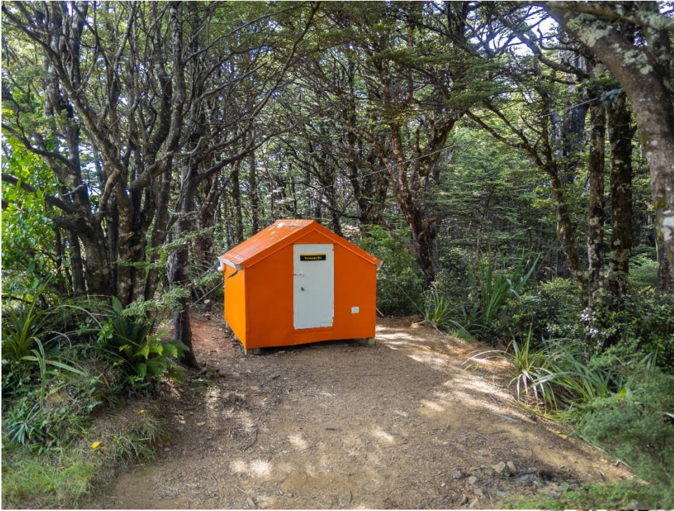
Figure 1 – Newly painted Taruarua Biv
